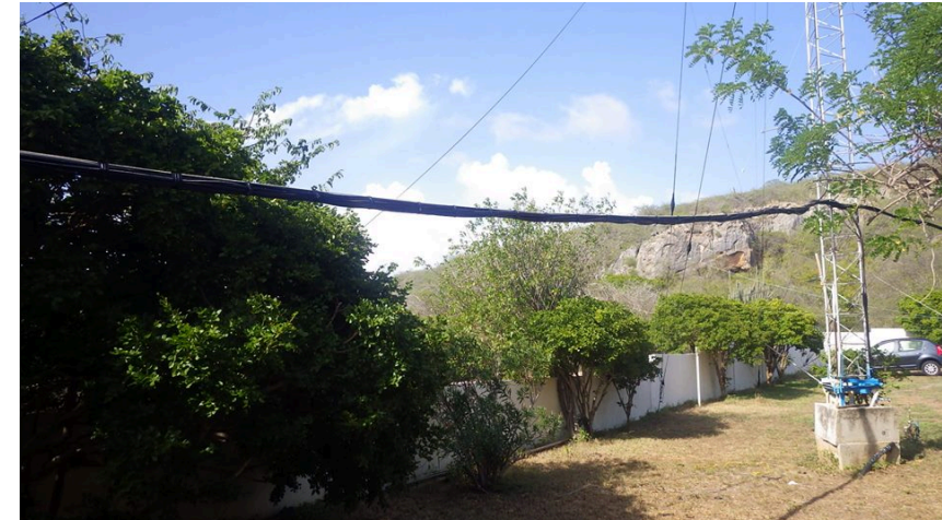
Finished. This used a lot of material and time!! But it will outlast all of us. The original messenger was 3/16 inch only and was not coated prior to installation. This is a much better, permanent fix
