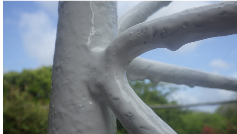
Fresh paint on the US/JA tower.
