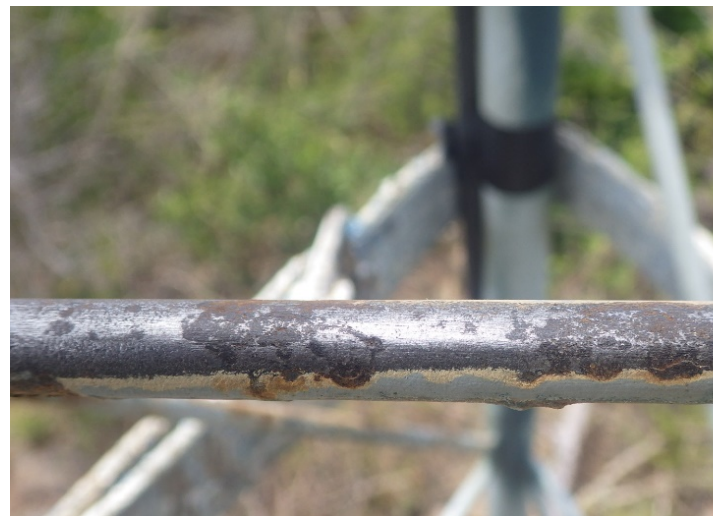
Cross-bar prepared for new paint.
