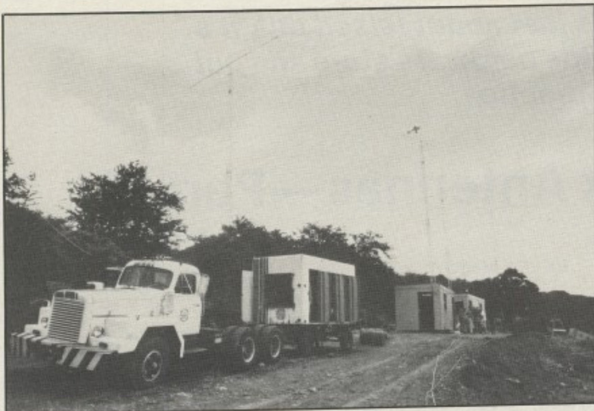
The 300 KW mobile generator being trucked to the operating site.
